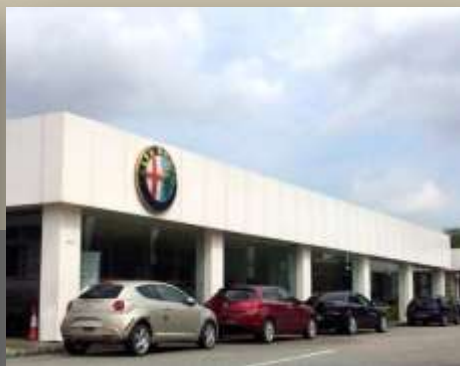
30 Teban Gardens Crescent
