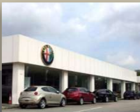
30 Teban Gardens Crescent
