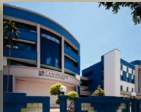
511 & 513 Yishun Industrial Park
