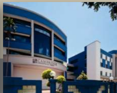
511 & 513 Yishun Industrial Park
