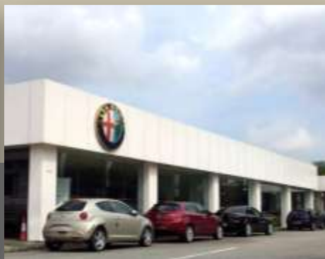
30 Teban Gardens Crescent
