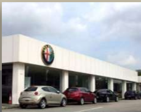
30 Teban Gardens Crescent
